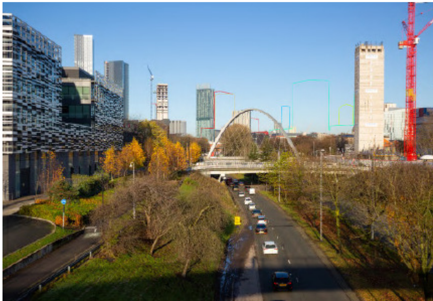
View 10 - an elevated footbridge over Princess Road
