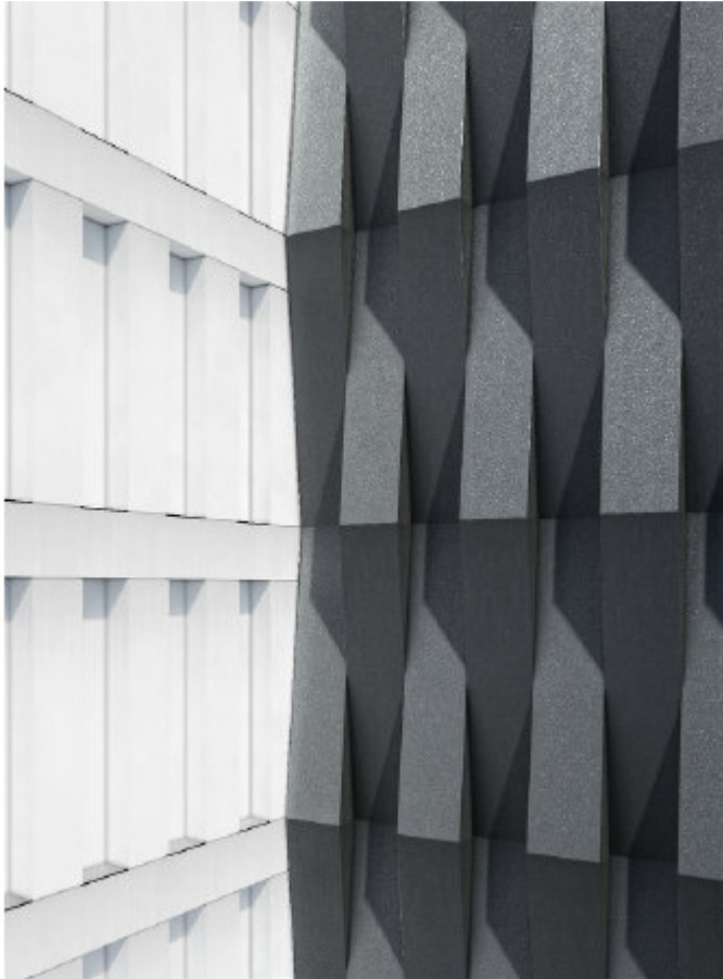
Extruded façade treatment (north façade)
