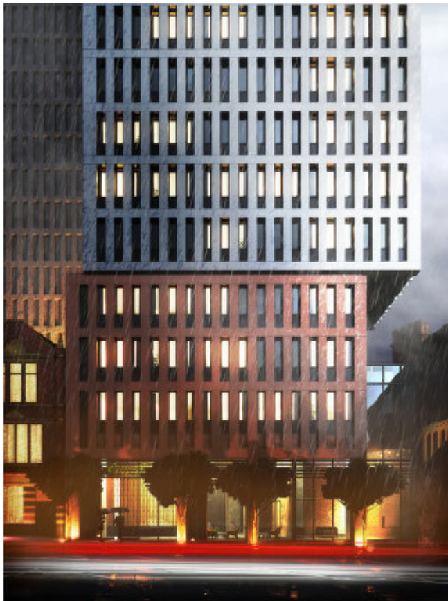
Base of the building from Deansgate including main entrance to Aparthotel
